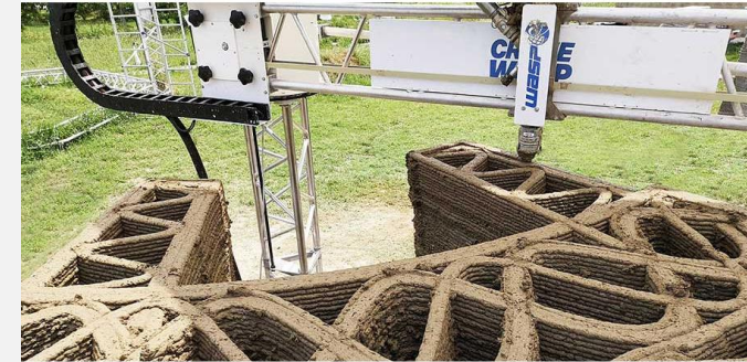
3D printed “earth walls”
